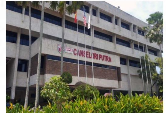
2) Chancellery Putra building, UPM
